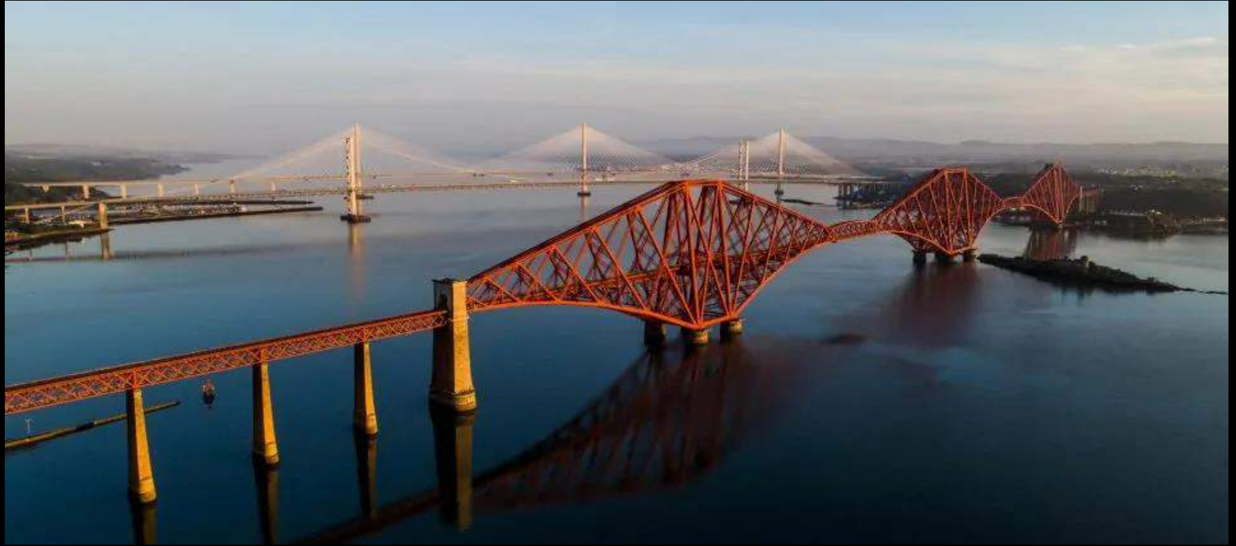
Edinburgh Rail and Road Bridges
