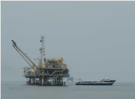
Exxon LNG platform in Mobile Bay, USA. August 2014
